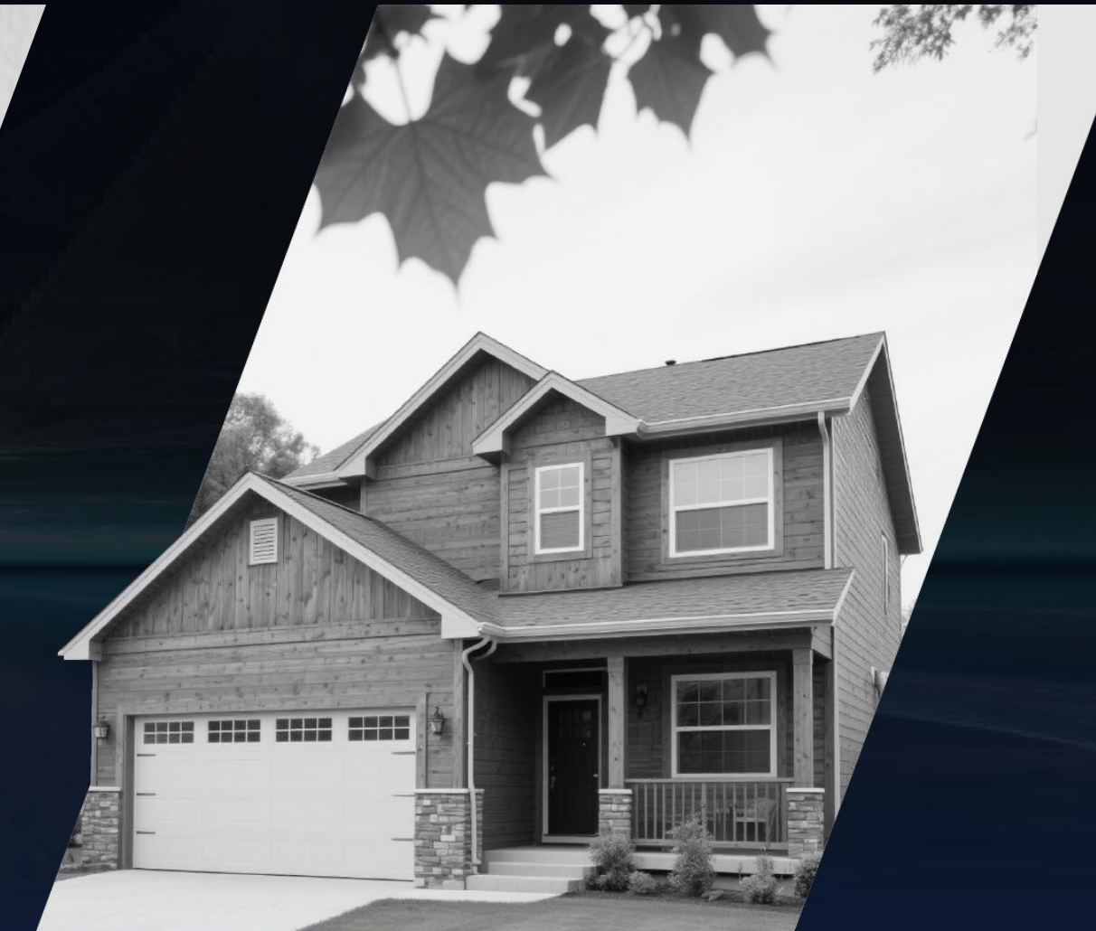
Vibration and Unusual Noise Transmission of Wooden Walls
